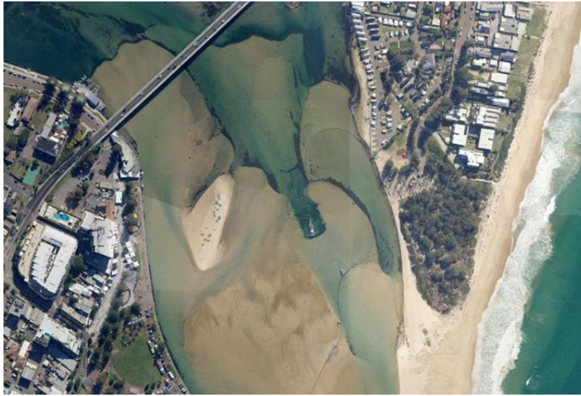
Figure 1.1: Dredging of tidal shoals at Tuggerah Lakes entrance in 2018. Source: NSW Spatial Services.
