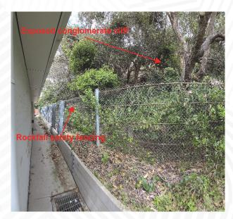
Photograph 6: Caves Beach picnic area, exposed conglomerate with rockfall protection from bushland and safety fencing, photographed January 2021.
