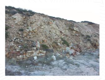
Photograph 9: Ongoing spalling and rockfall from old fill platform at Middle Camp Beach, Catherine Hill Bay, photographed 2015.
