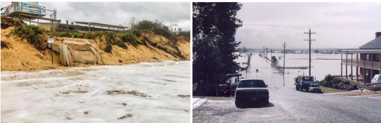
FIGURE 3-3 EROSION AT UMINA BEACH IN 2015 (LEFT) AND 1986 FLOOD AT WINDSOR (RIGHT)
