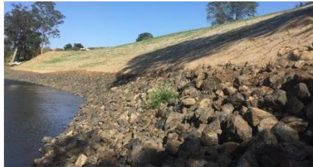
**Scour protection** – Structural bank protection (i.e. rock) armour the underlying sediments and protect them from fluvial and wave action.
