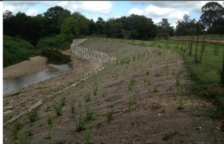
**Geotechnical stability** – Reducing the bank slope can increase the geotechnical slope stability.
