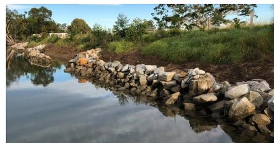
Figure 25. Example of rock fillet bench protection in the Kalang River
