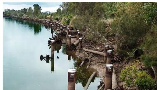
Figure 24. Example of timber fillet bench protection in the Coomera River (photo: City of Gold Coast)
