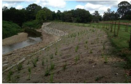
**Hydraulic roughness** – Structural works provide frictional resistance which dissipates flow energy and reduces the near bank velocity and shear stress. Timber structures have a reduced design life and may not be appropriate for providing long-term protection to high-value built assets.
