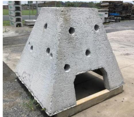
Figure 23. A concrete pyramid habitat reef unit (photo Catchment Solutions)
