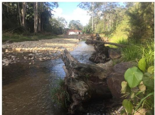
**Figure 27.** Instream timber toe protection
