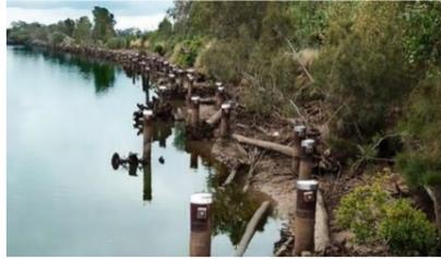
**Hydraulic roughness** – Structural works provide frictional resistance which dissipates flow energy and reduces the near bank velocity and shear stress. Timber structures have a reduced design life and may not be appropriate for providing long-term protection to high-value built assets.
