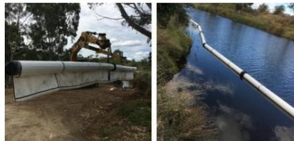
**Wave and scour protection** – A floating boom can dissipate the wave energy and protect the bench and lower bank from wave action.
