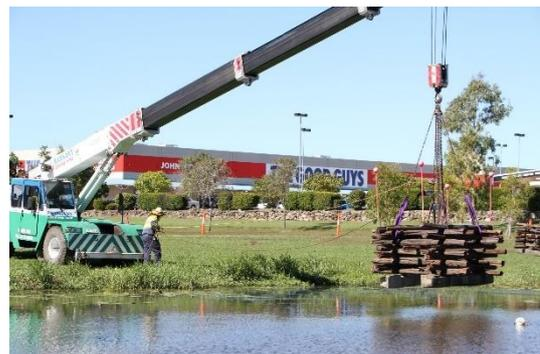
**Figure 28.** Modular complex timber structures (photo Catchment Solutions)
