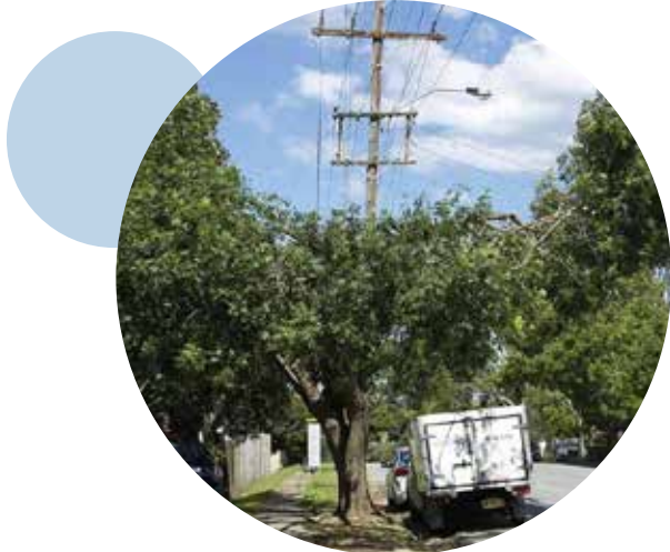
Poor Tree Selection/ Conflicts with overhead power-lines
