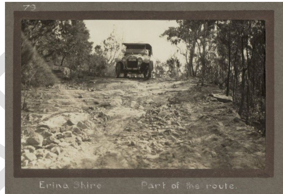
Figure 6.3 Part of the route of the Peats Ferry Road (Pacific Highway) within the Erina Shire. 1920s. (Source: MHNSW, State Archives Collection FL116227 79)
