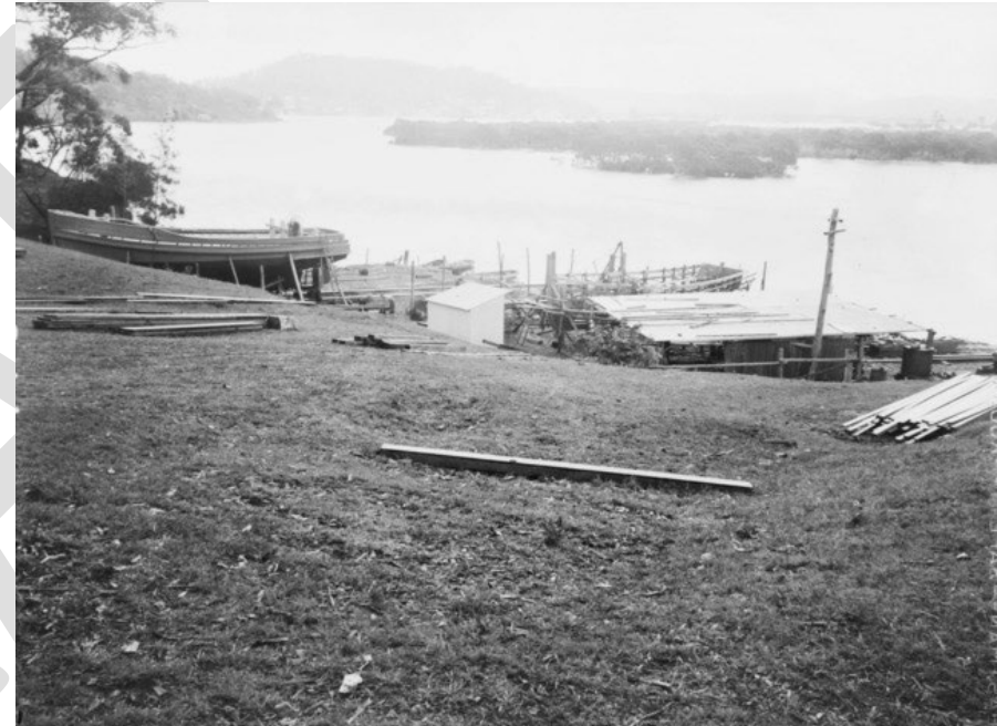
Figure 5.7 Section of the Palermo shipyard near Empire Bay, October 1943. (Source: Australian War Memorial, 069752)
