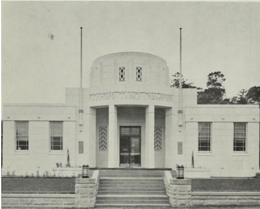
Figure 8.15 New Council Chambers, Gosford, 1939. (Source: Building , 24 May 1939, p 2)
