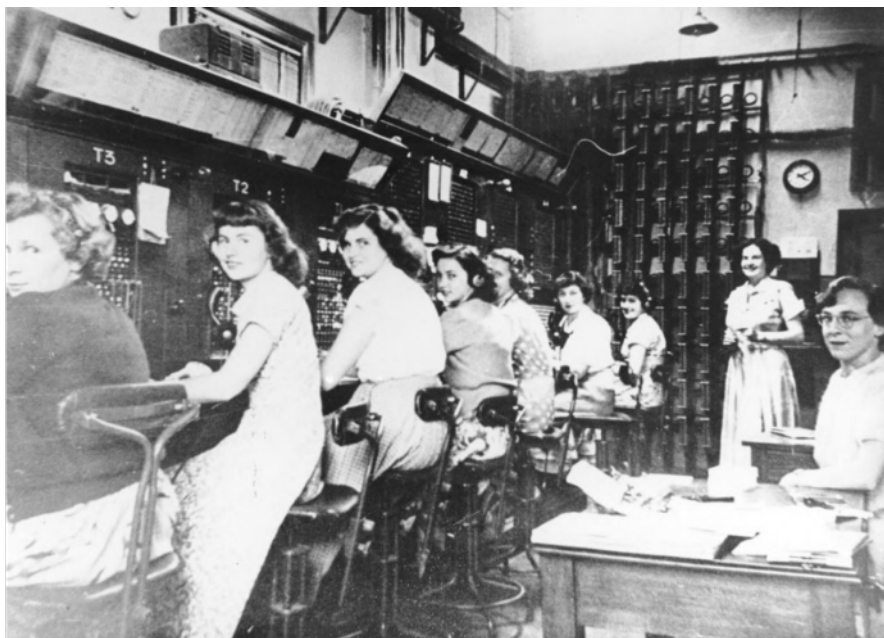
Figure 6.22 Telephone operators, Gosford Telephone Exchange, c1950s. (Source: Central Coast Library Service)
