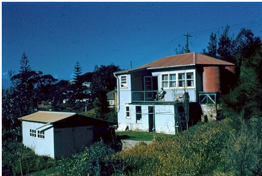
Figure 9.13 Les Collinge's house at Avoca Beach, 7 June 1960. (Source: Gostalgia, local history from Gosford Library)
