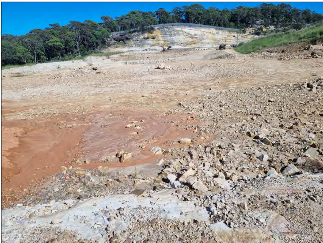
Photo C.2 View of the project site (looking west) showing the reworked surface devoid of topsoil
