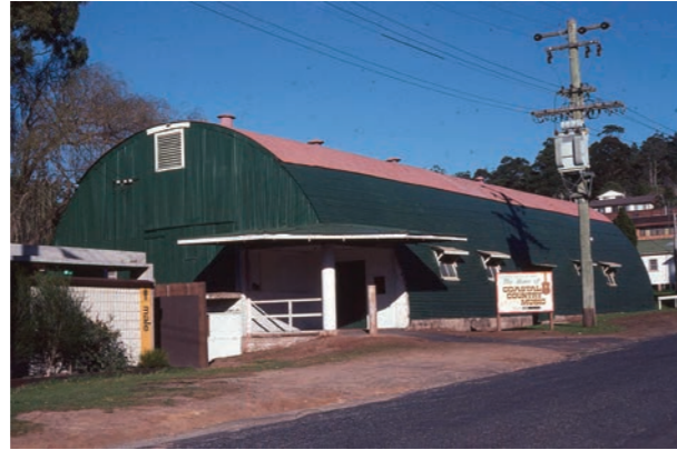
Public toilet block was built in 1979
