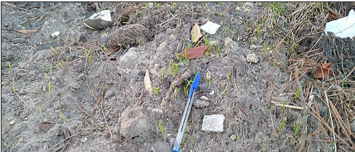
Figure 8: Fragments of potential asbestos containing material observed on the ground surface.
