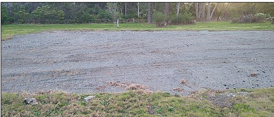
Figure 6: Former tennis court filled with a sandy gravel.
