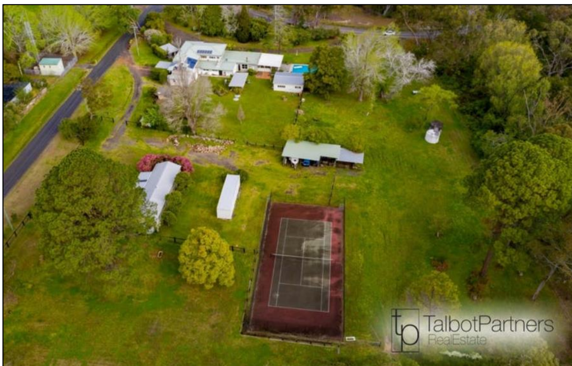
Figure 3: Site layout prior to demolition of structures (source: TalbotPartners RealEstate).
