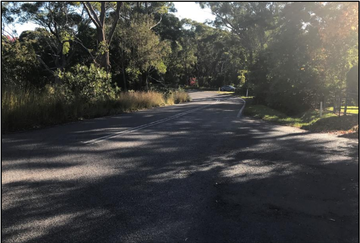
Photo 2 – View to right for driver exiting Ashbrookes Road.
