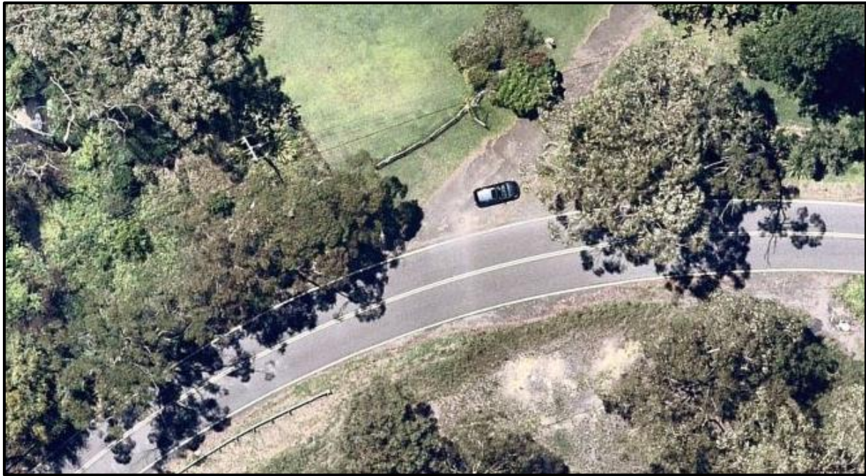
Photo 4 – Aerial photo showing existing alignment for driveway on the Pacific Highway to allow for direct access for northbound traffic
