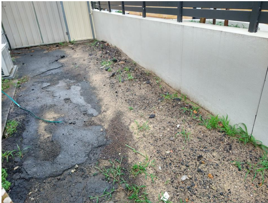
Photo 3 – Western side of Ettalong Beach Motel
