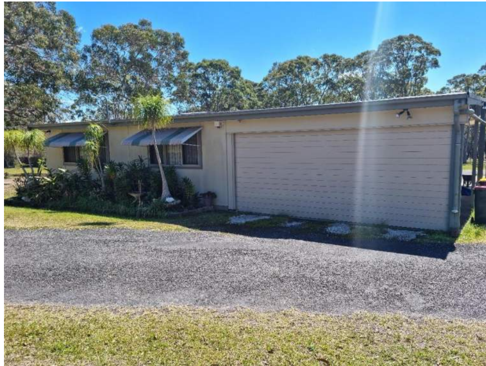
Photo 1: Residential dwelling located on Lot 27 (semi-rural property).
