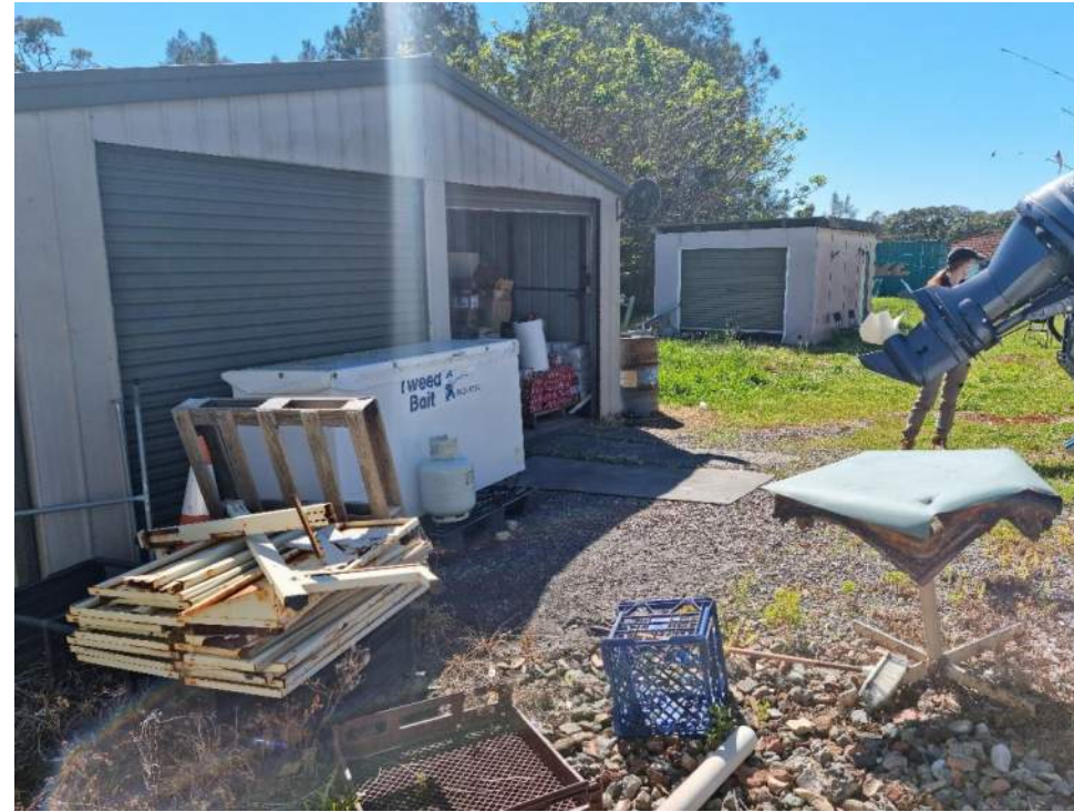
Photo 38: Third shed onsite holding general inventory/stock for the BP shop. This shed is in relatively good condition.
