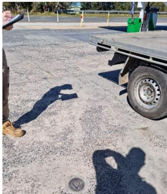
Photo 28: Monitoring well located on the eastern side of the service station.
