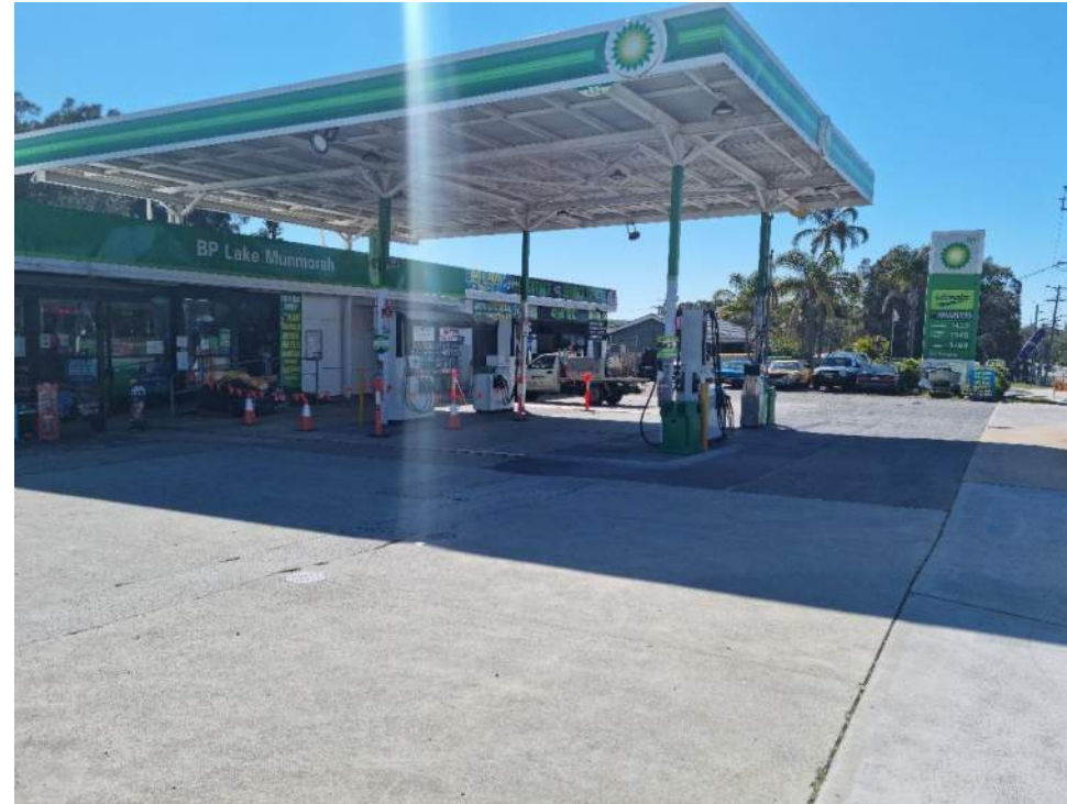
Photo 26: View of Lot 12 (BP service station) from the footpath adjacent to the Pacific Highway, showing the main BP shop building, adjacent garage service centre and the four bowsers of the service station.
