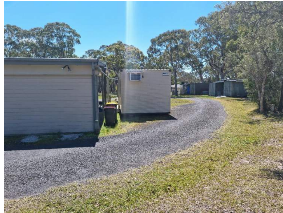
Photo 2: Detached demountable building adjacent to the garage on Lot 27.
