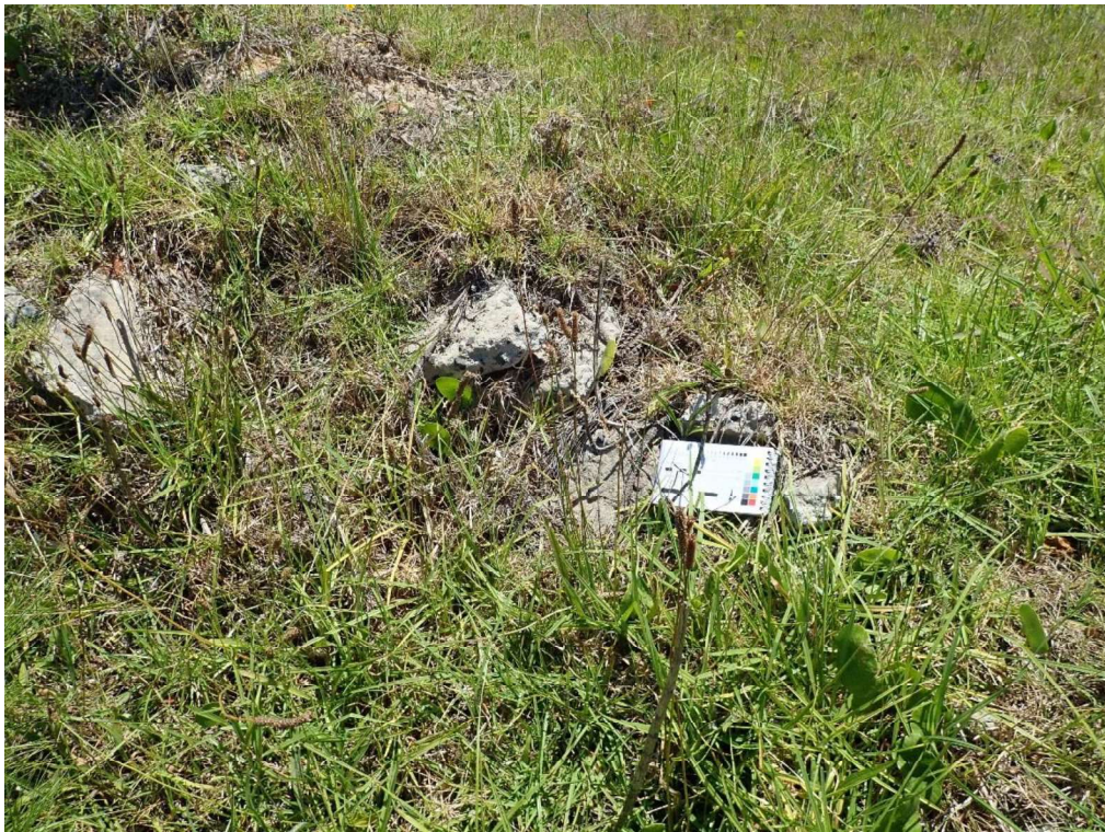
Photo 11 – Showing crushed concrete north west corner No. 295
