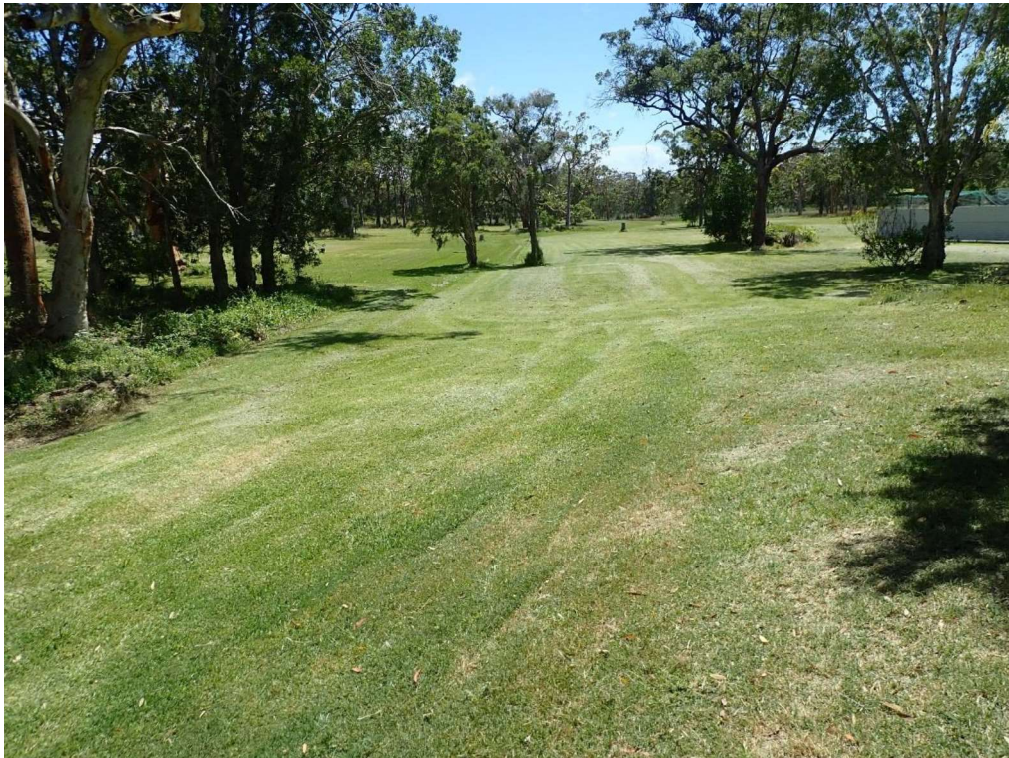
Photo 18 – Looking north down No. 305 the darker green grass generally indicates the drainage flow path
