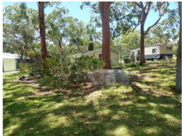
Photograph 24. Block 305 looking east, buildings from left to right include workshop, main residence (background), cattery, relocatable building.
