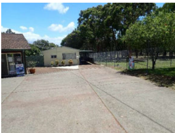
Photograph 17. Block 305 looking north along eastern boundary toward original dwelling on site. Note recent concrete pour for drainage works.
