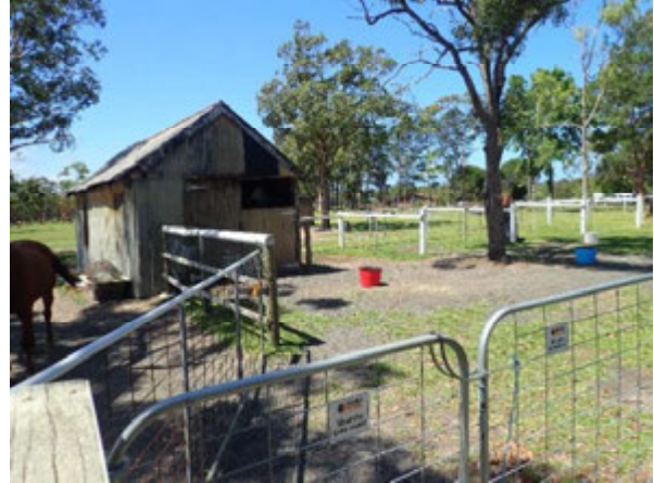
Photograph 2. Block 285 looking north east at the shed to rear of main residence.
