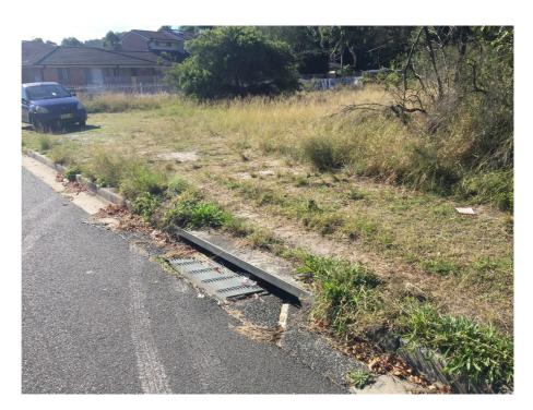
Figure 3 – Photo: Sag Kerb Inlet Pit at site road frontage (MacLeay Avenue)
