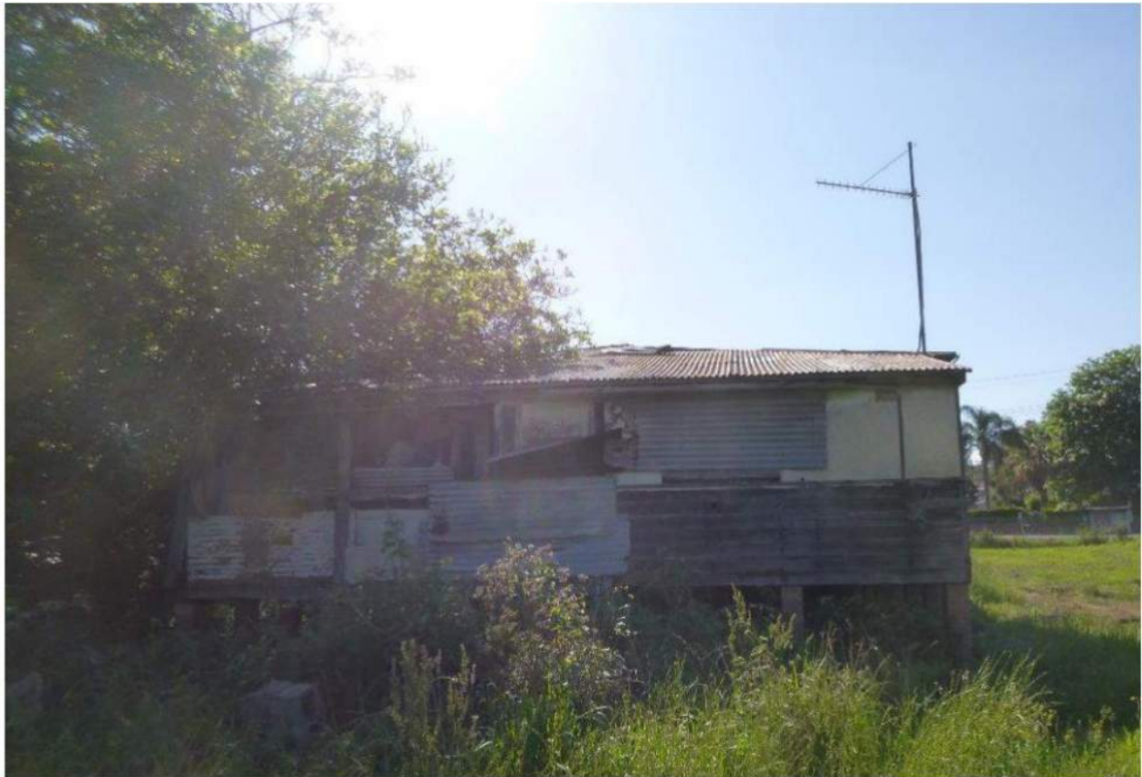
Photograph 3: Abandoned Residential Dwelling (see OIN 4 on Figure 2 in Appendix A).
