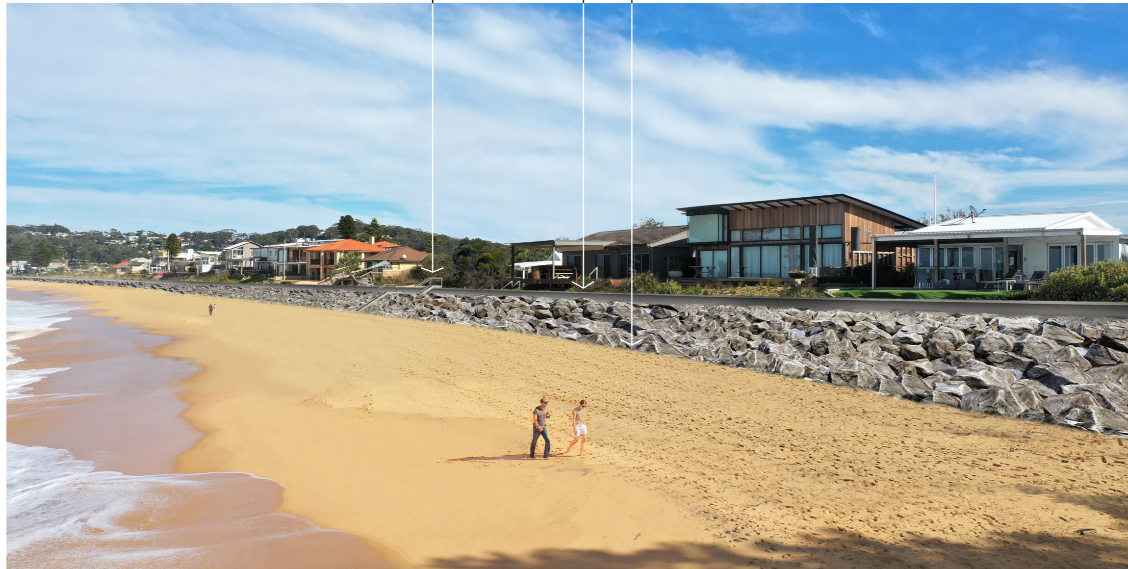
image: concept design option 1 - basalt rock revetment (Wamberal Terminal Coastal Protection Assessment, Draft Final Stage 3 - Seawall Concept Design Options, May 2021)
