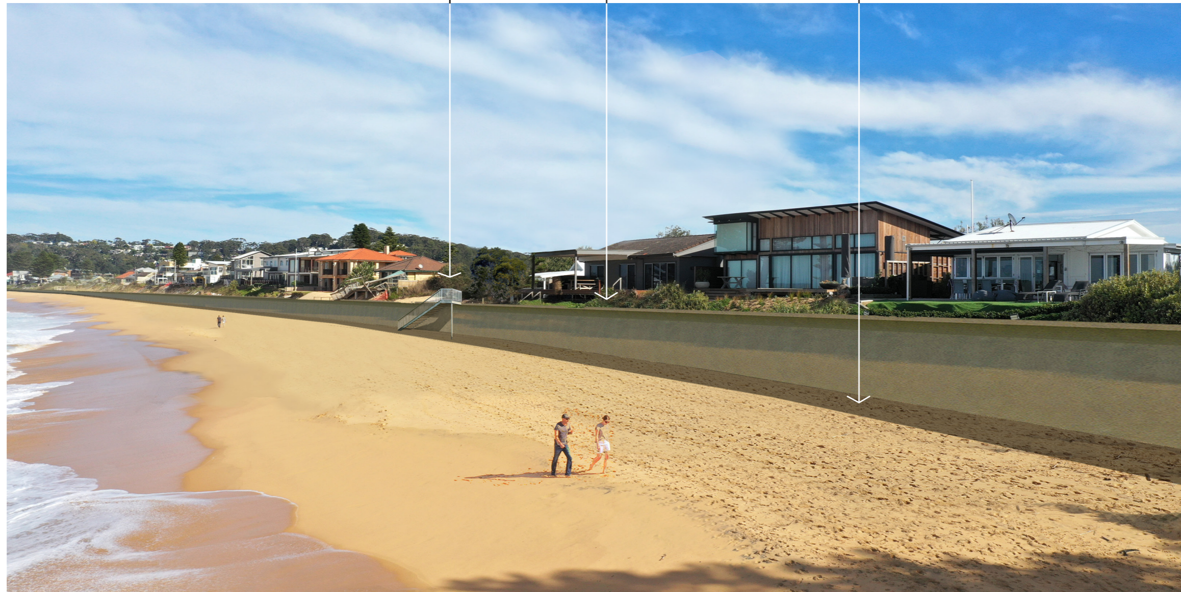
image: concept design option 3 - vertical seawall (Wamberal Terminal Coastal Protection Assessment, Draft Final Stage 3 - Seawall Concept Design Options, May 2021)
