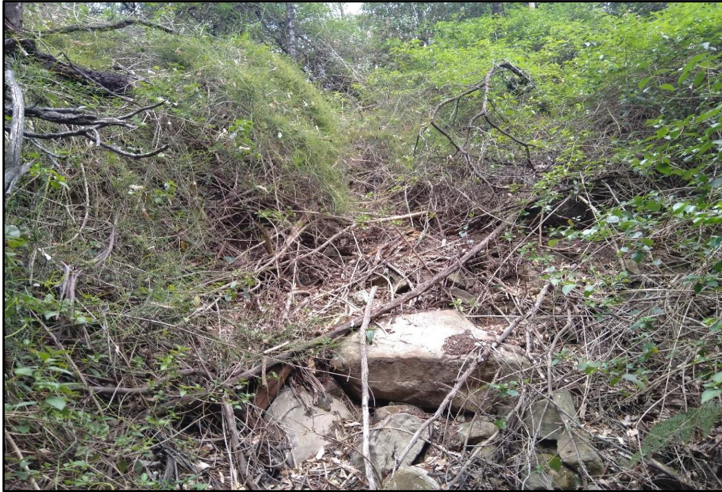
Photo 21: View of sandstone boulders at base of cutting, at western end
