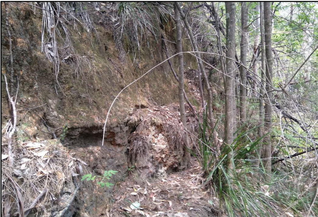
Photo 20: Example of loose soil wedge
