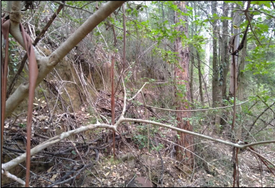
Photo 19: View of cutting looking west
