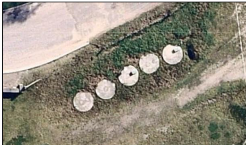
Plate 16 Wastewater Treatment Tanks – Function Centre
