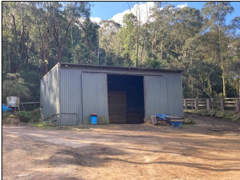
Plate 7 Hay Shed and Above Ground Fuel Storage
