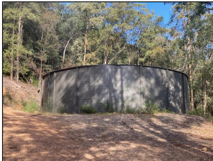
Plate 22 Water Storage Tank
