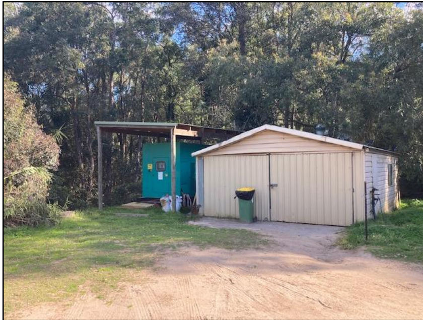
Plate 9 Shed and Back-Up Generator
