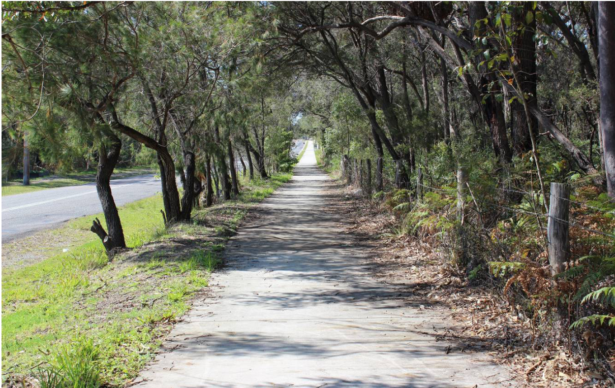
Photograph 8 – Off-road cycle / pedestrian path in Mulloway Road adjacent to the site.
