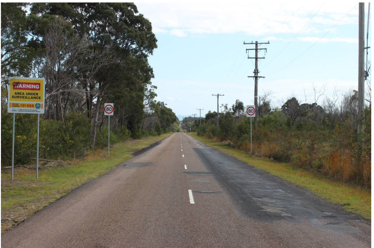
Photograph 5 – Chain Valley Bay Road in the vicinity of the Pacific Highway
