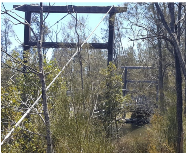
Photo 6: Karignan Creek Footbridge
