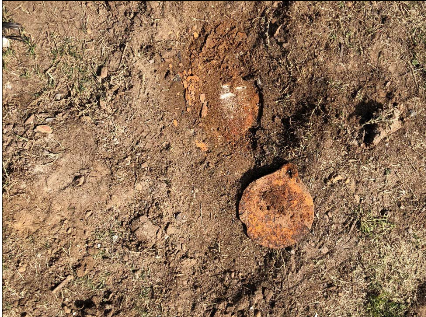
PHOTOGRAPH 20: PORTION 7 - CONCRETED DIP POINT FOR UST AT FORMER SERVICE STATION
