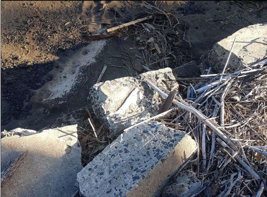
PHOTOGRAPH 11: PORTION 3 – CONCRETE USED AS FILL MATERIAL WITHIN SEA WALLS
