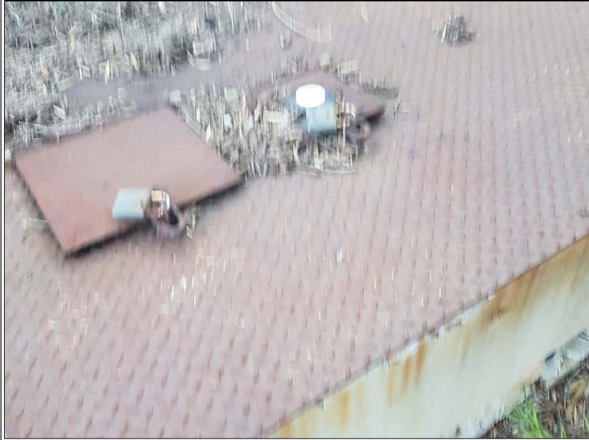
PHOTOGRAPH 2: PORTION 1 – AST NORTH OF LAUNDRY BUILDING
