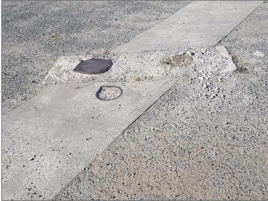
PHOTOGRAPH 20: PORTION 7 - CONCRETED DIP POINT FOR UST AT FORMER SERVICE STATION
