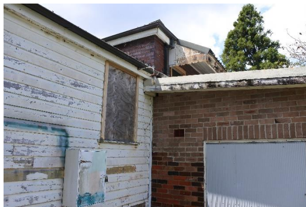
Figure 87 – View of west elevation, original eaves evident.
