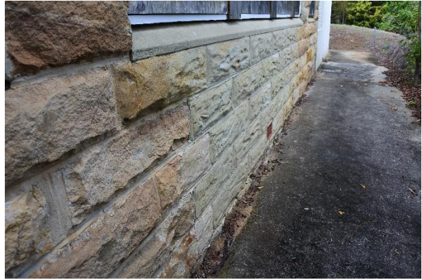
Figure 23 – Detailed view of concrete 'stone look' infill on north elevation.
