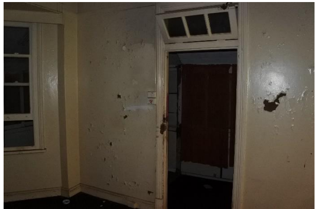
Figure 97 – View of original external doorway leading to northern enclosed verandah in central room.
