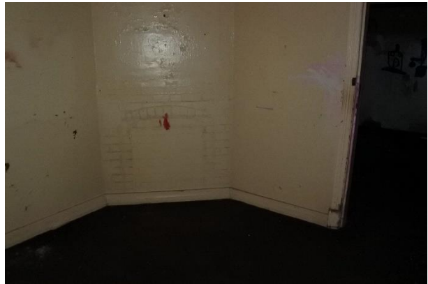
Figure 95 – View of bricked up fireplace within central room.
