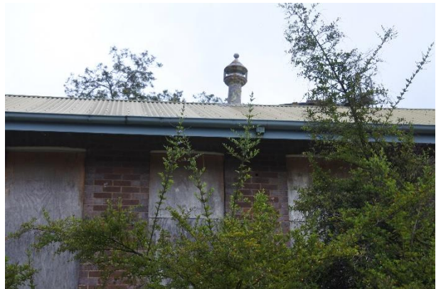
Figure 33 – Detailed view of ornate ventilation crown.
