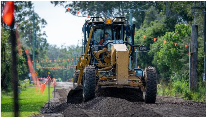
Image: Final reinstatement of the pipeline route.
