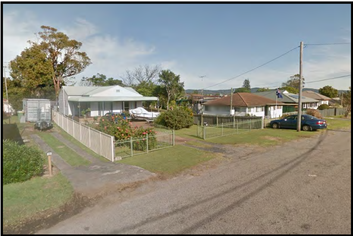
Plate 28 A typical location along Elsiemer St with no kerb and gutters.
