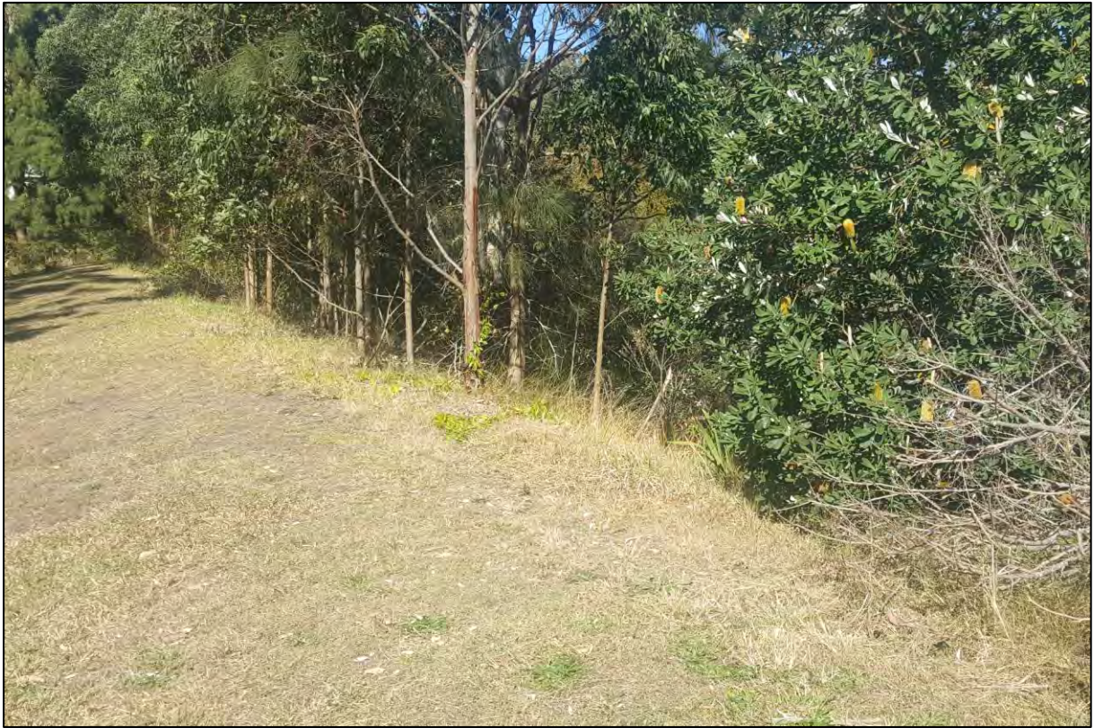
Plate 2 Example of significant trees/vegetation along the downstream embankment of Basin A
