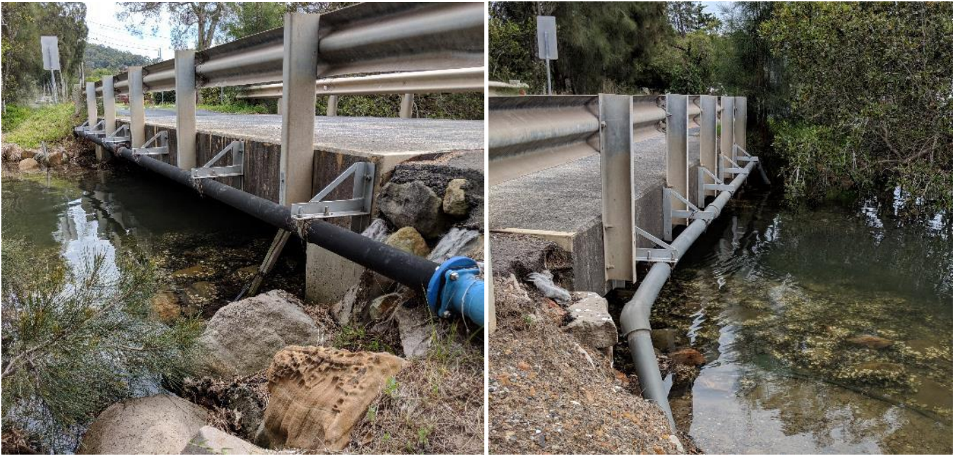
Davistown – Morton Crescent bridge downstream / upstream
