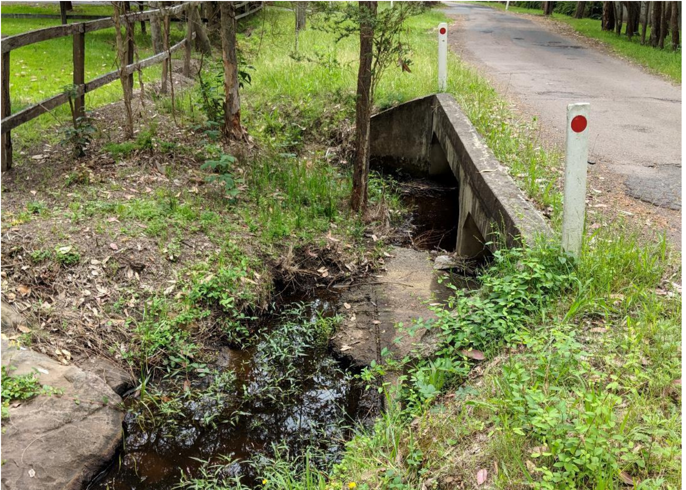
Empire Bay – twin box culvert crossing on Pomona Road
