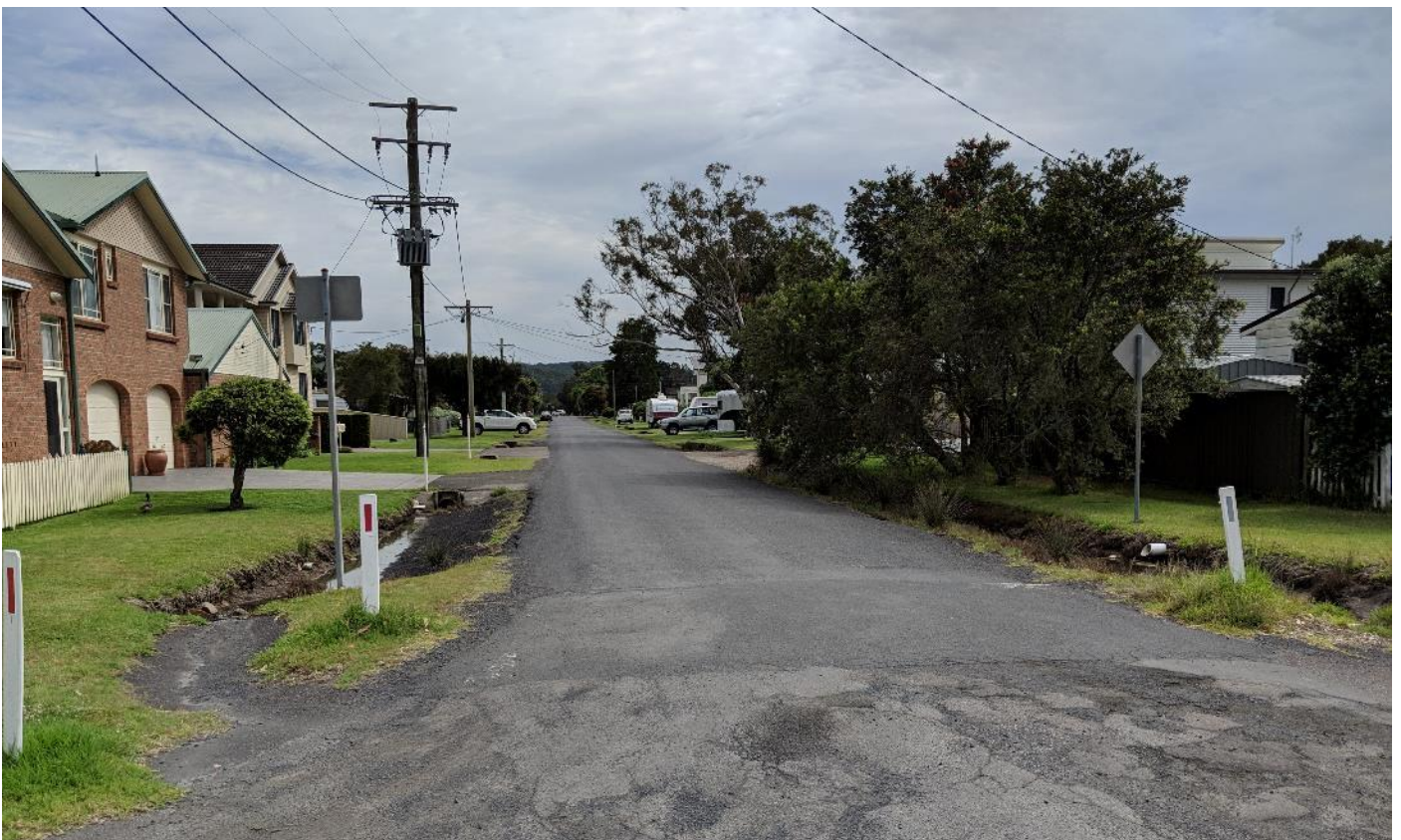
Davistown – south end of Pine Avenue
