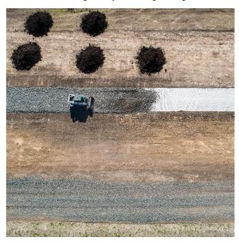
Image: Reinstatement works along the pipeline route
