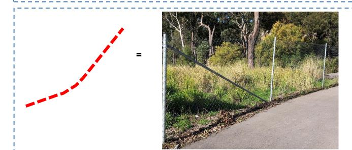
The southern boundary of the playspace will be fenced using 1.8 metre chain wire fencing to deter public access into the protected areas. Fencing will connect to existing fencing along the eastern side of Fairwater Drive.
