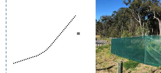
The existing 1.8 metre chain wire fencing with green mesh will be removed from the front of the playspace and replaced with 1.2m high playground fencing to separate the playspace and traffic travelling along Peninsular Drive.
