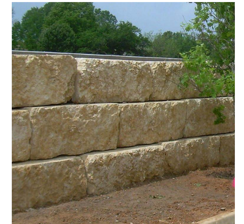
SANDSTONE LOG RETAINING WALL
