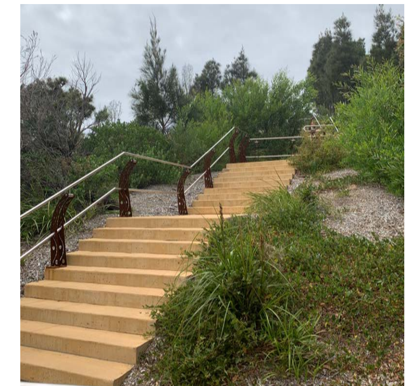
COLOURED CONCRETE STAIRS AND WALKWAY
