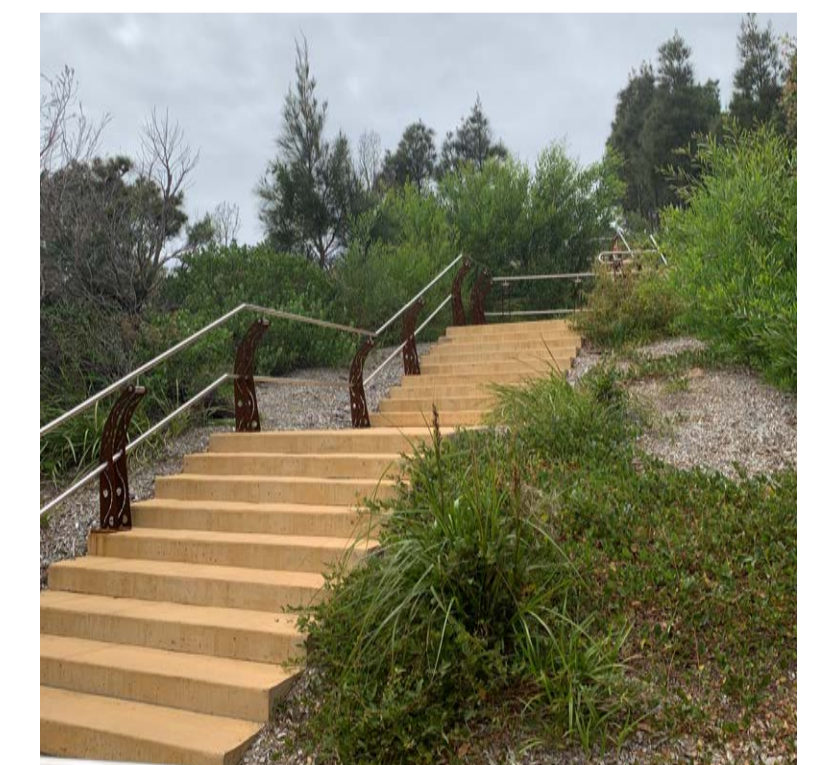
COLOURED CONCRETE STAIRS AND WALKWAY
