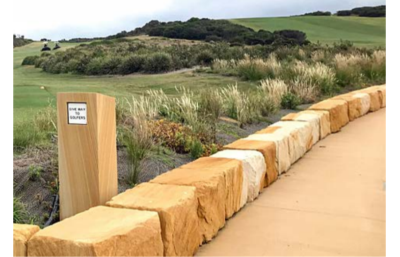
SANDSTONE LOG RETAINING WALL
