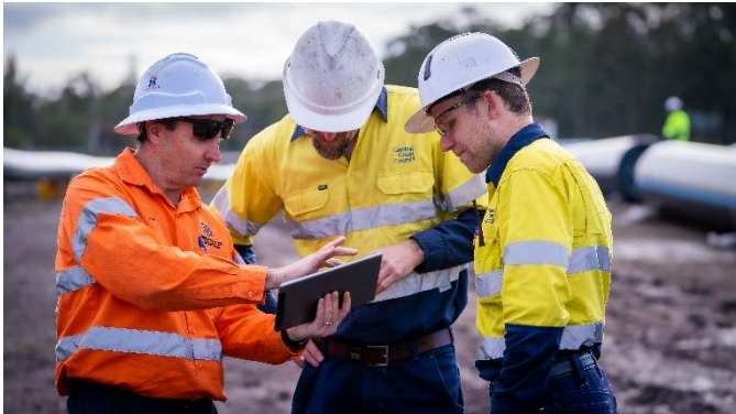
Image: Central Coast Council staff and contractors onsite inspecting works at Mardi
