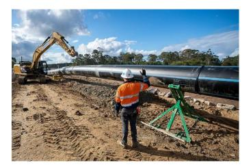
Once the pipe has being unloaded along the construction corridor, the pipes are joined by a welding process. This involves clamping the ends of the pipe together then applying high temperature hot steel plates to melt the two ends of the pipe bonding them and creating a high strength butt weld. The water pipeline is then fully buried, by excavating a trench 1.6 metres wide and up to 4 metres deep in some locations.
