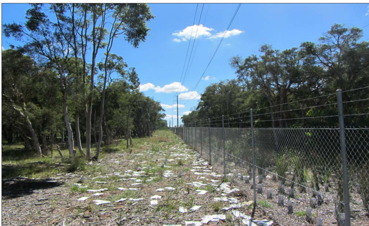
Plate 1 Vegetation hazard and Powerline easement east of the site
