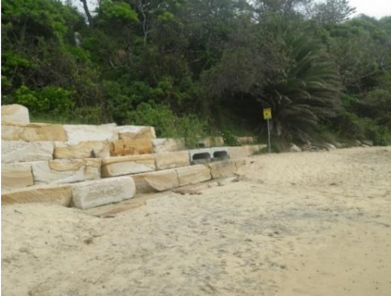
Figure 7 - Wall and vegetated slope in Domain 1
