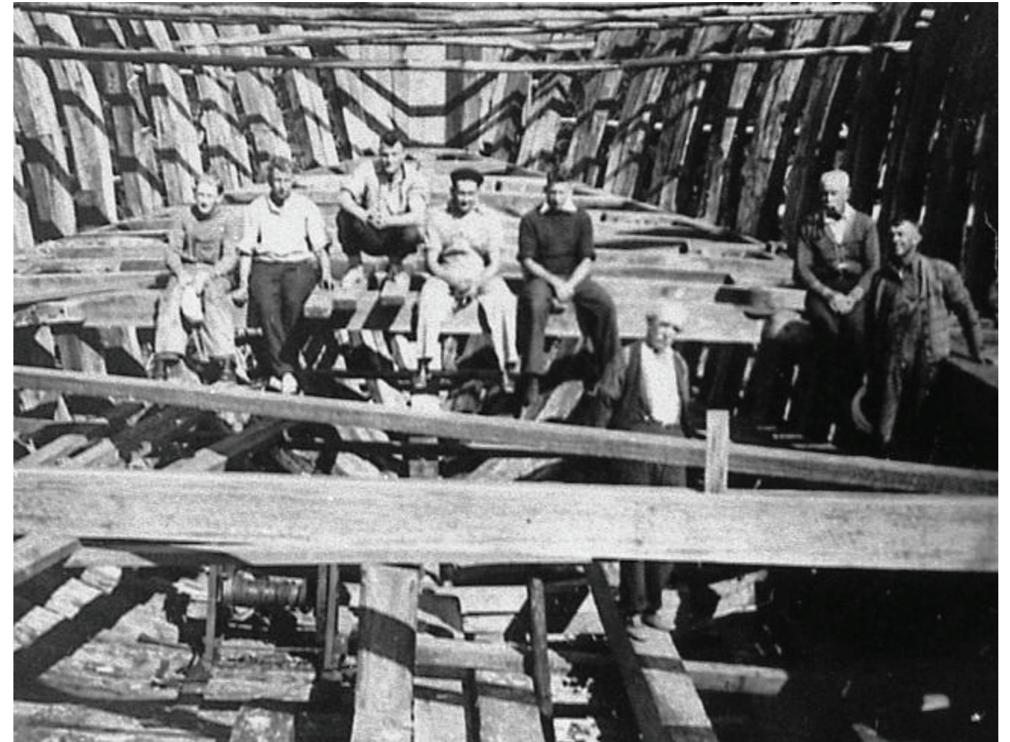
Shipwrights at work on the Patricia Cam at Beatties shipyard, Daleys Point. Source: Gosford City Council
