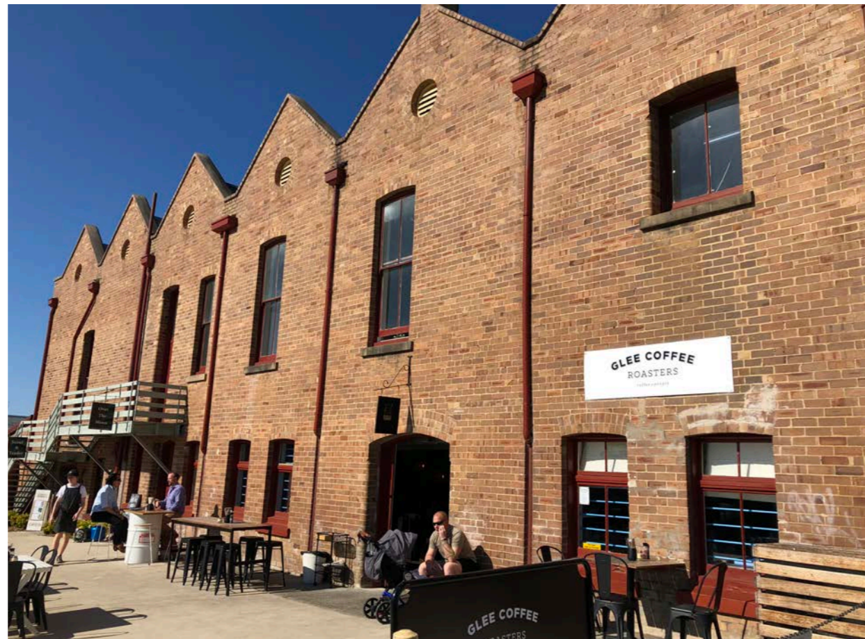
Chapman building, Wyong
