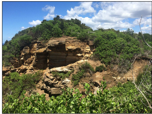
02 VIEW FACING SOUTH-EAST AT THE PROPOSED LOCATION FOR THE WALKWAY BRIDGE CROSSOVER
