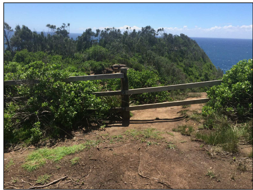
01 VIEW FACING NORTH-EAST AT THE PROPOSED LOCATION FOR THE WALKWAY BRIDGE CROSSOVER
