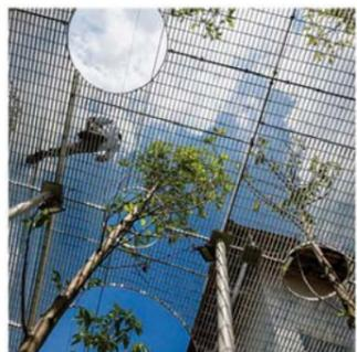
Grated flooring on the viewing platform will allow users to view the water below, while ensuring sunlight can still reach the seabed. The options of aluminum, weathered steel or fibreglass will be decided in detailed design stages.
