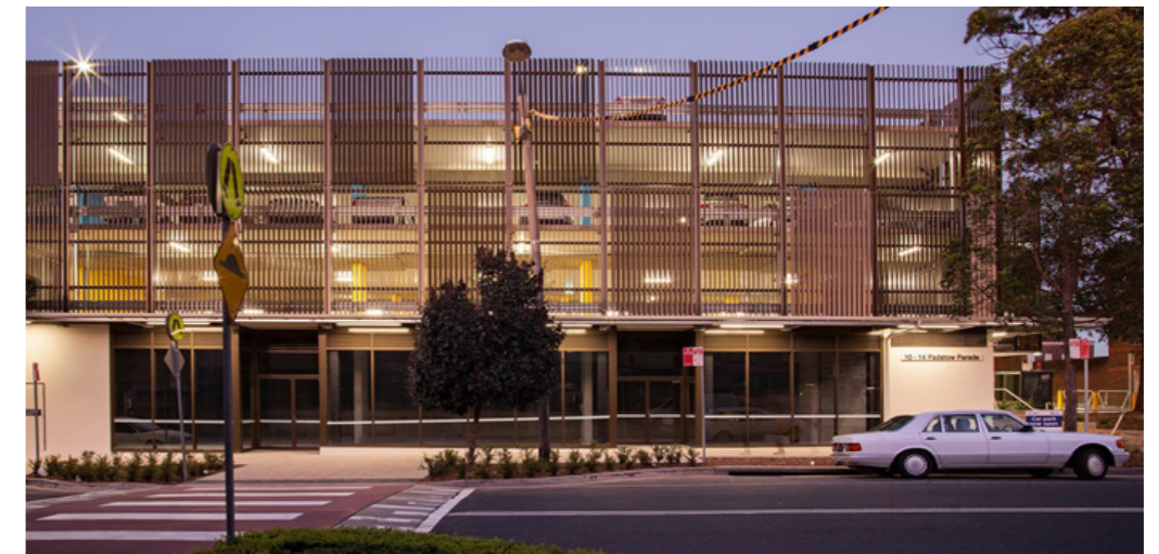
Padstow commuter car park, NSW (image: AW Edwards)
