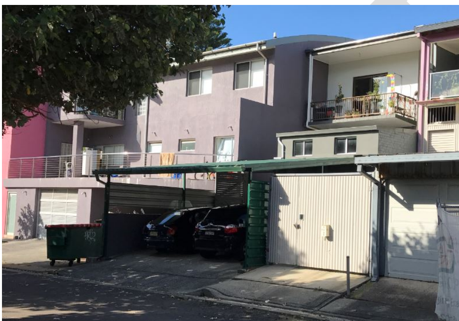
Figure 12 Example of service areas provided off laneways and not visible from the main street
